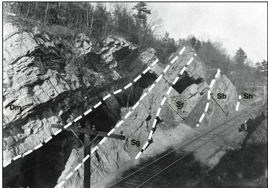
**Figure 13.** Annotated photograph of a cut along the rail trail, near Fourth Lake, showing the west limb of the Hickory Bush anticline, and the remnants of abandoned roof and pillar cement quarries. The photograph was taken by G. van Ingen, before reforestation, and was reprinted by Osborn (1921).
