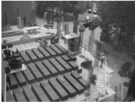
Fig. 4. The "bathtubs," forms for the underside of the floors.
