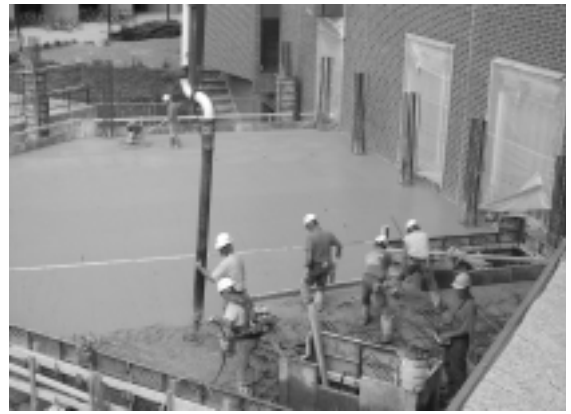
Fig. 5. Concrete mixed at ground-level was delivered overhead via lengthy piping. Pouring the floors was a real team effort.
