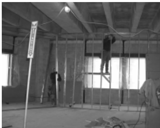
Fig. 9. With winter here, window openings are covered by plastic and workers frame in corridor walls.
