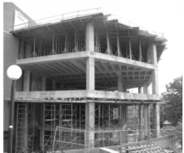
Fig. 6. Early fall. Temporary plywood decking for the fourth floor is in place and the decking between the second and third floors has been removed.
