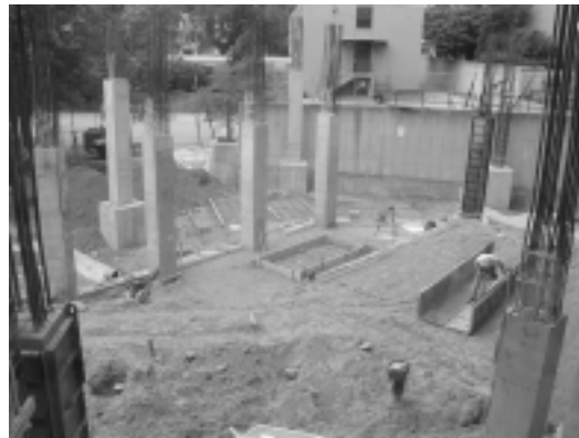
Fig. 3. Concrete and rebar support beams were constructed in stages.
