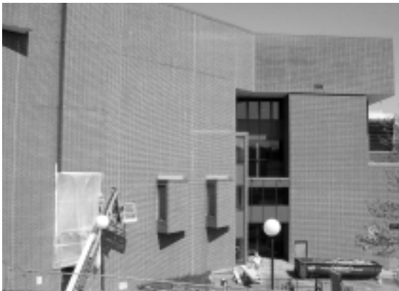
Fig. 1. Late summer: first floor window wings were removed from the south side of Weeks I.
