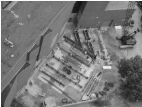
Fig. 2. The loading dock was removed and foundations poured.
