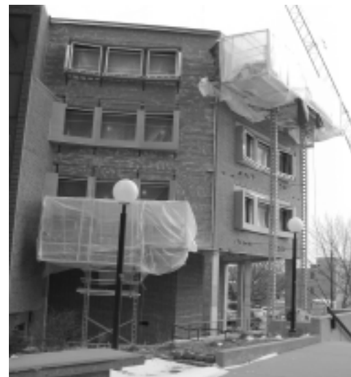
Fig. 8. December, the west face. Bricklayers are working in heated scaffolding. The new brick matches that on Weeks I and II.
